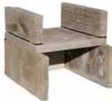
Step 8 - Install floor firebrick
