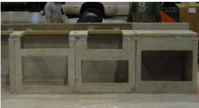
Step 7 - Mark and cut appliance openings to specifications of appliance manufacturer, using construction marker and standard masonry saw blades.
