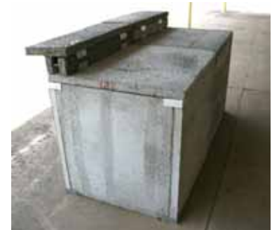
Step 6 - Place top panels and backsplash kits, if applicable. Shown with bar top backsplash.
