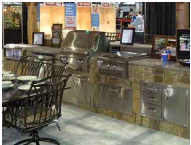
Finished installation of unit shown at left.
