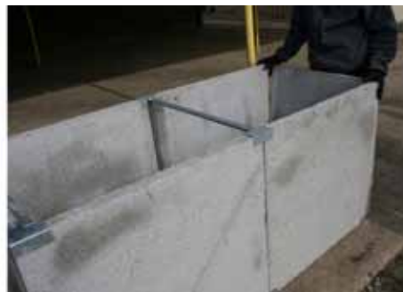
Step 5 - Place end panel and final end bracket.
