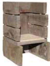
Step 8 - Install floor firebrick
