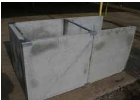
Step 4 - Continue raising side panels, using Sonolastic® adhesive and brackets.
