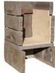
Step 9 - Add firebrick to walls
