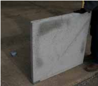
Step 4 - Continue raising side panels, using Sonolastic® adhesive and brackets.
